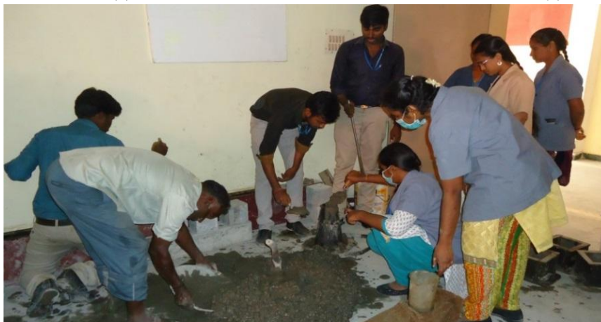
(d) Conducting slump test and casting of beams
