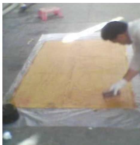
Fig.2 Application of resin over the fibre
